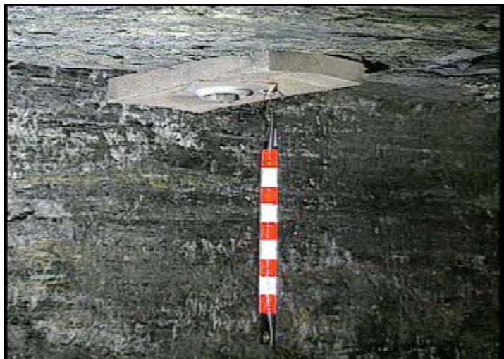
Figure 2. Reflector Marking Last Row of Roof Bolts
