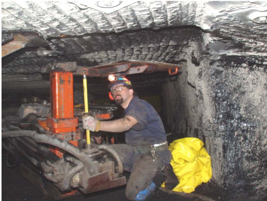
Figure 7. Drilling a Roof Bolt Hole
