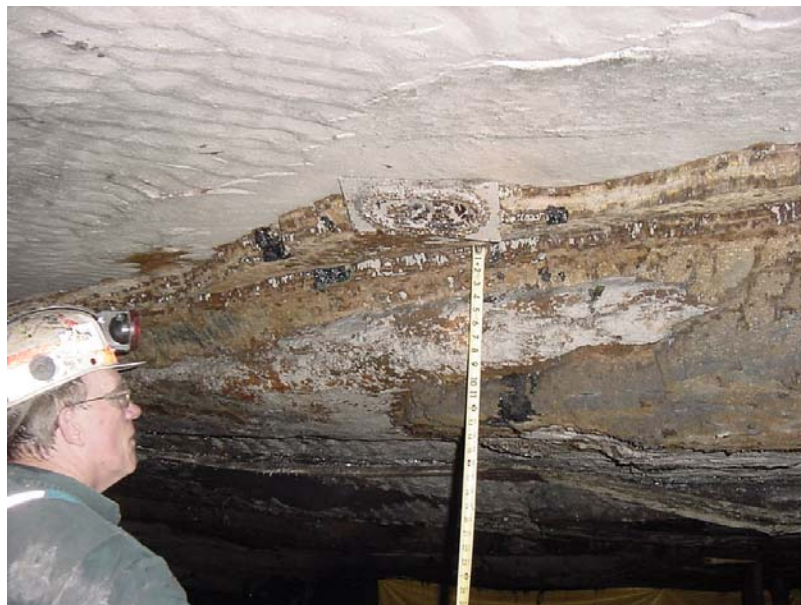
Figure 1. Variable Roof Rock – Sandstone, Shale, and Coal Interspersed
