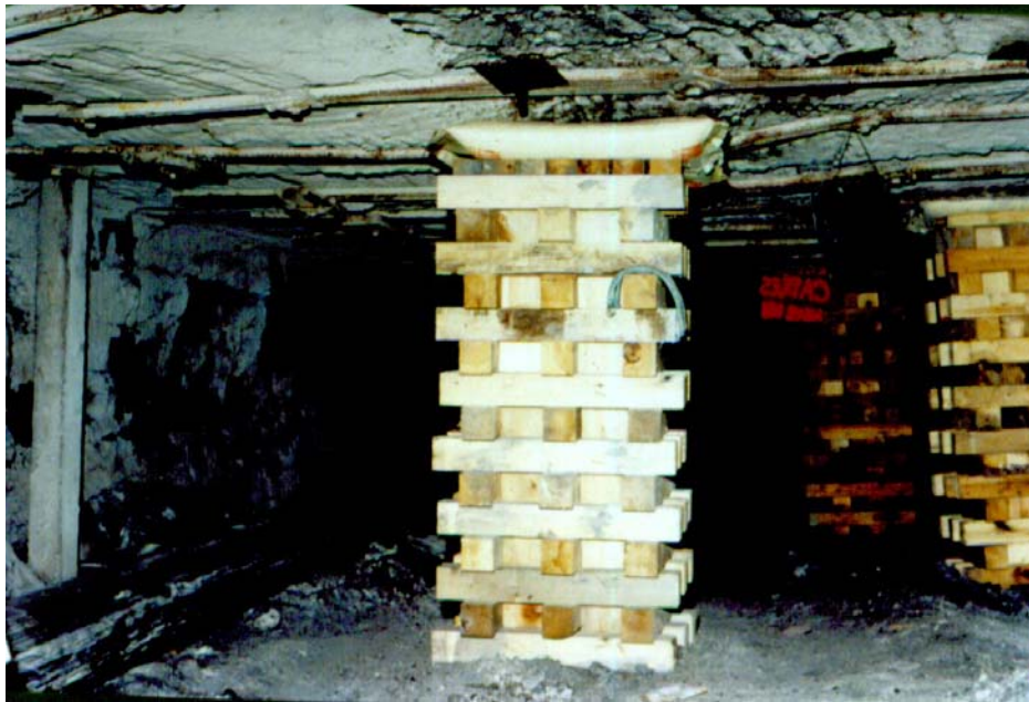
Figure 8. An “Engineered” Wood Crib
