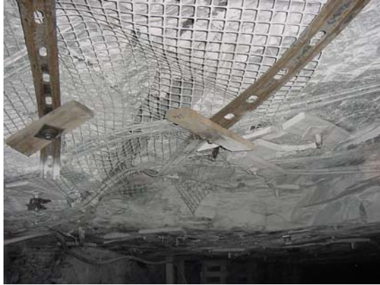
Figure 6. Intersection With Supplemental Roof Support
